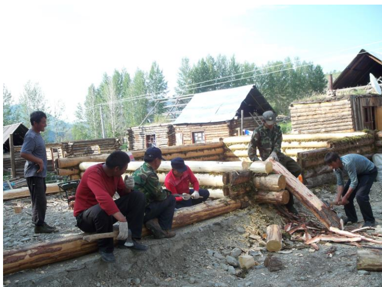
Tuva people in China building traditional wooden houses (Courtesy: Yuxin Hou)
