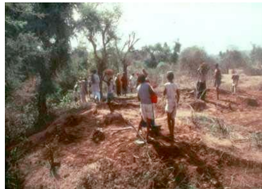
Photo: Vivek Gour-Broome Construction of an earthen dam by the villagers
