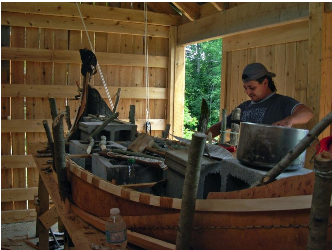
Charles (Chuck) Commanda, a traditionally trained Algonquin canoe builder, constructs his canoes using traditional materials and techniques along with a few modern aids. © Peigi Wilson
