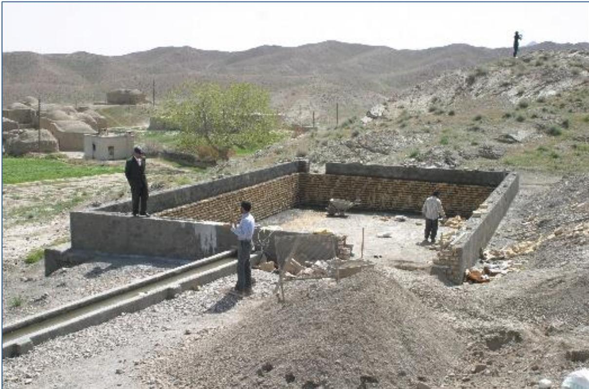
**Figure 1:** The restoration of a *qanat* and its open storage tank – a traditional water supply used in the customary rangelands of the Abolhassani Tribal Confederacy in Iran. Photo courtesy of Taghi Farvar / Cenesta.
