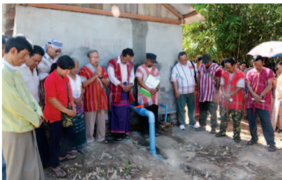
A prayer service was held after the gravity-flow water system was successfully installed
